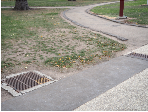
One of the problem drainage pits in the square
