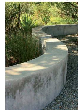
Concrete seat/ barrier
