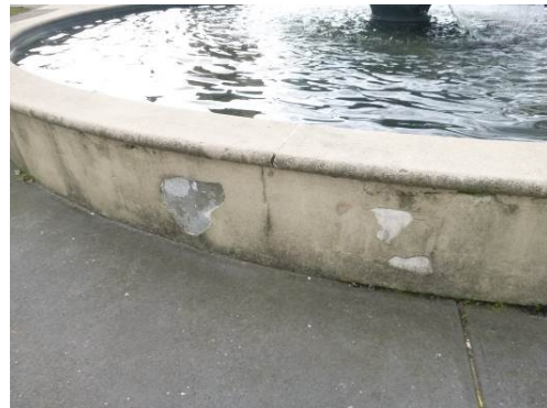
Cracks in the render of the fountain base wall
