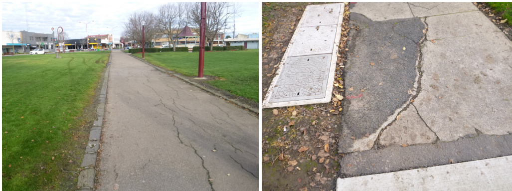
Existing cracks in the footpaths
