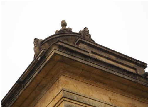
Discolouration in the top part of the memorial
