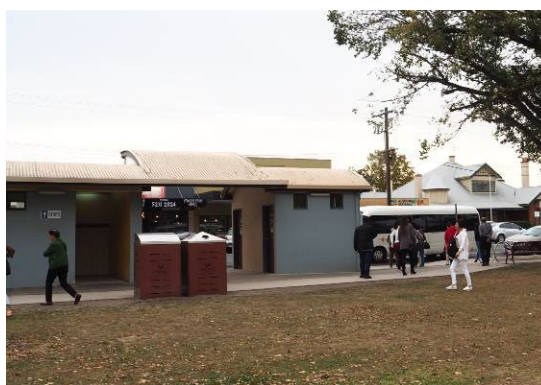
Existing public toilet facilities
