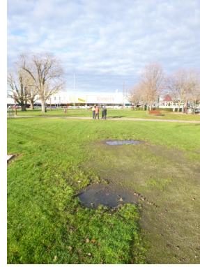
Existing local depression on the northern section
