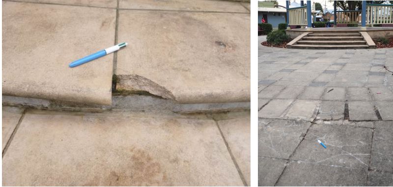
Masonry paving tiles to the Rotunda
